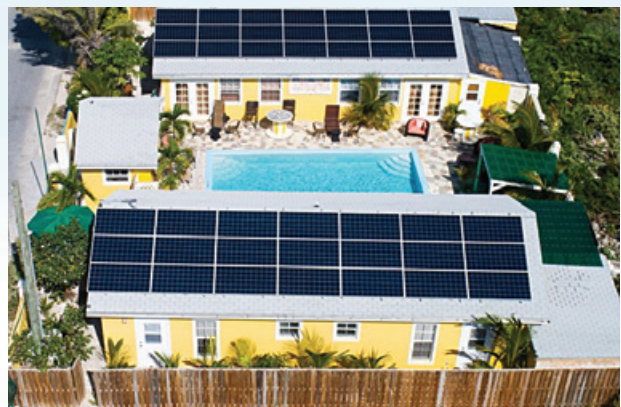
A FortisTCl UORE Program solar installation project in Grand Turk.
