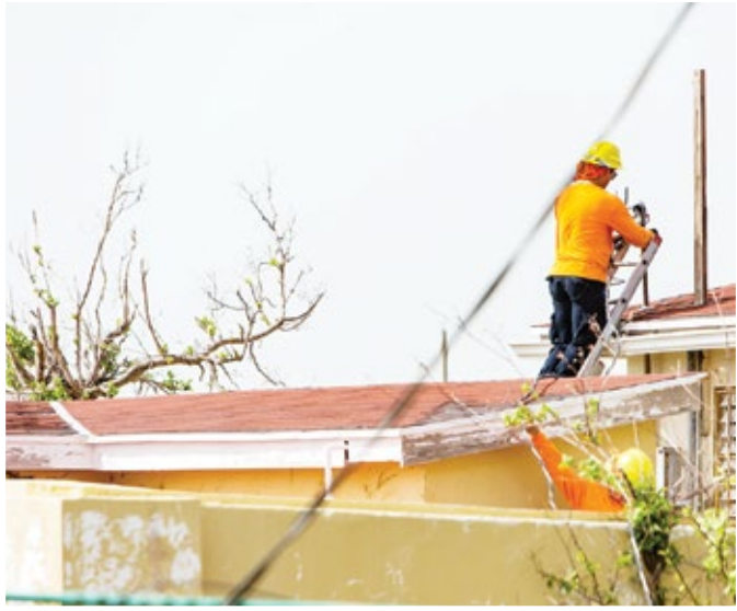
>> Crews at work, connecting homes with power on South Caicos.
