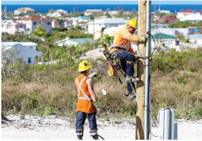
>> A view of restoration work on Grand Turk.
