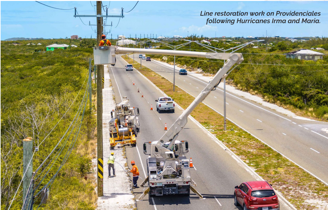
Mechanical Technician I Tarek Fulford performs maintenance work at FortistCI, Providenciales.
